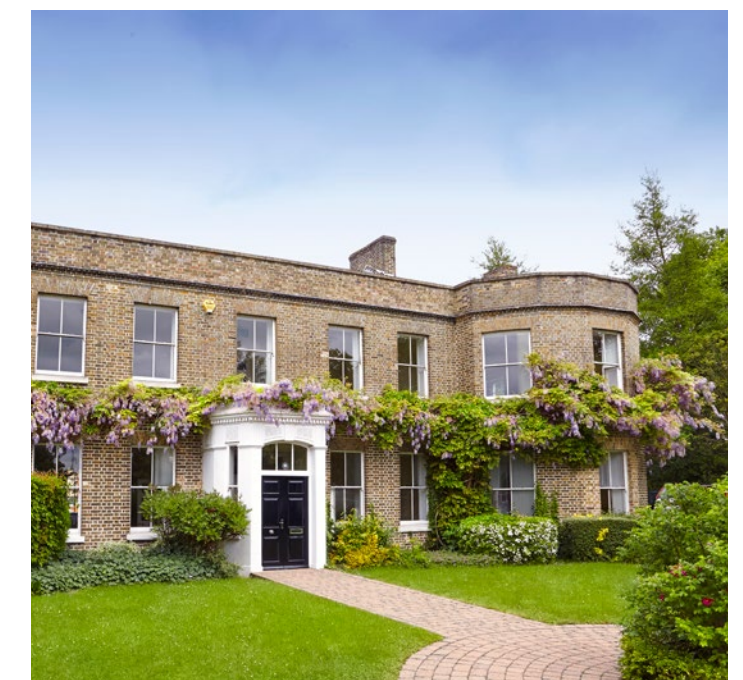
The Manor House – Royal Quay, Harefield
